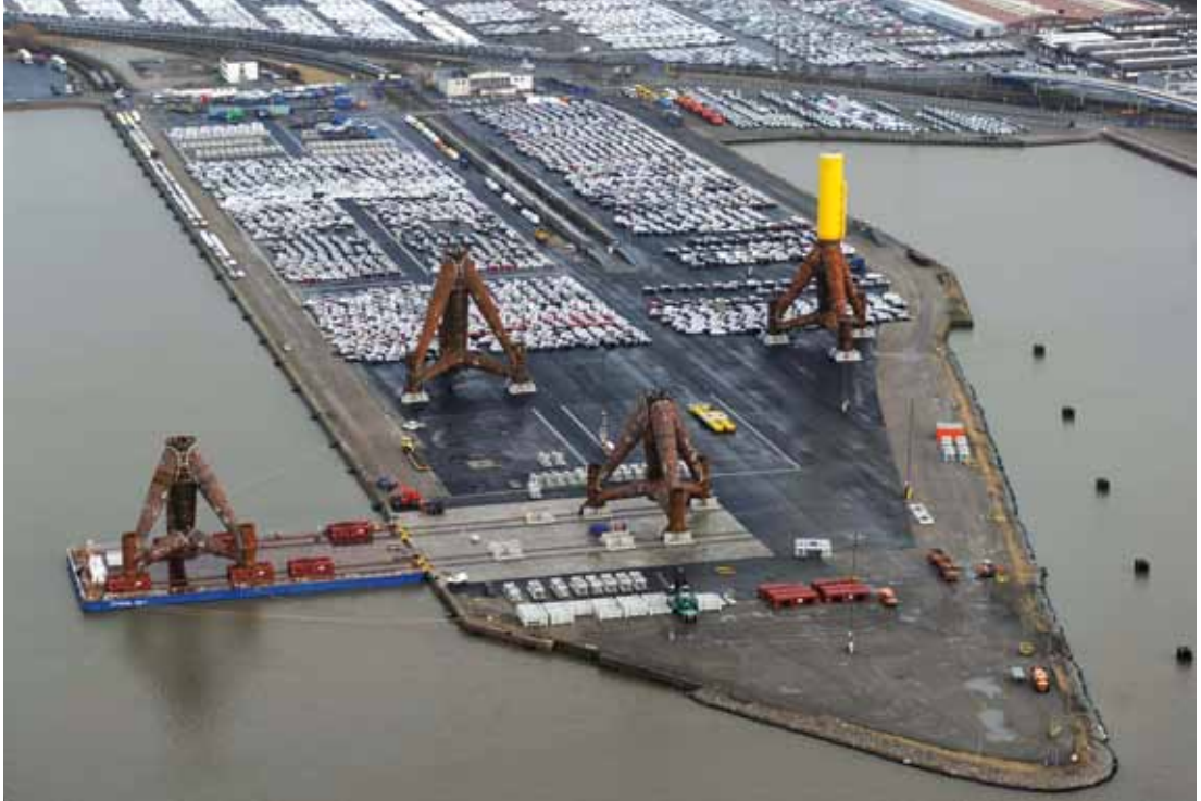
ABC peninsula in Bremerhaven with OFFSHORE BHV 1 pontoon
