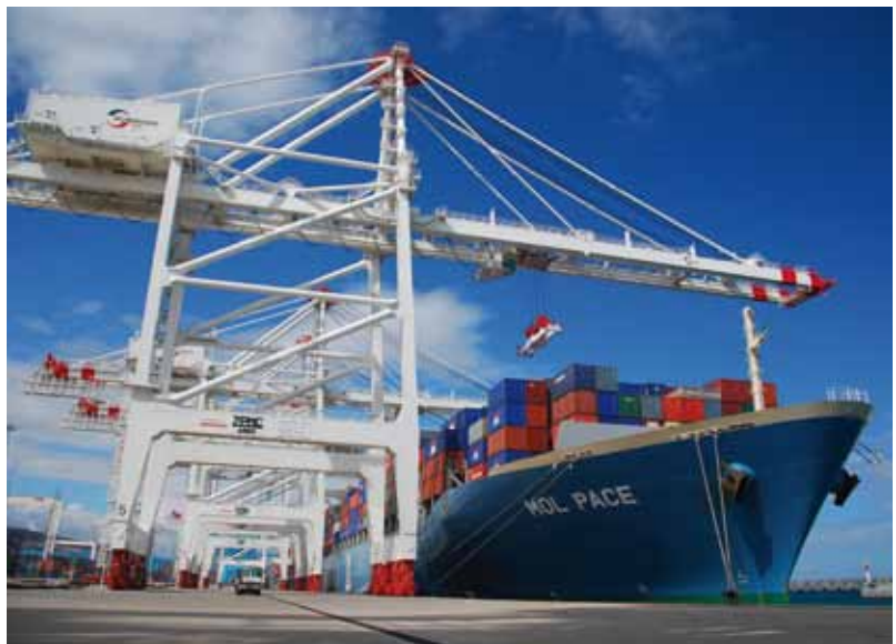
EUROGATE container terminal in Tangier, Morocco
