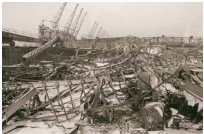
Destroyed shed 15 in Bremen's Überseehafen, 1941
