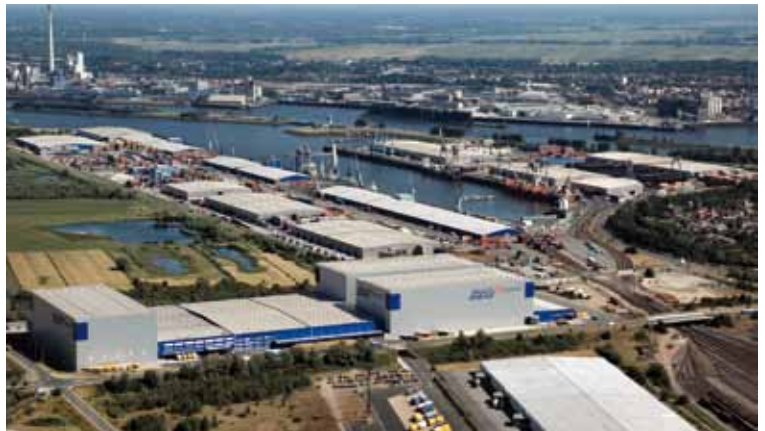
BLG high-bay warehouse and Neustädter Hafen, Bremen
